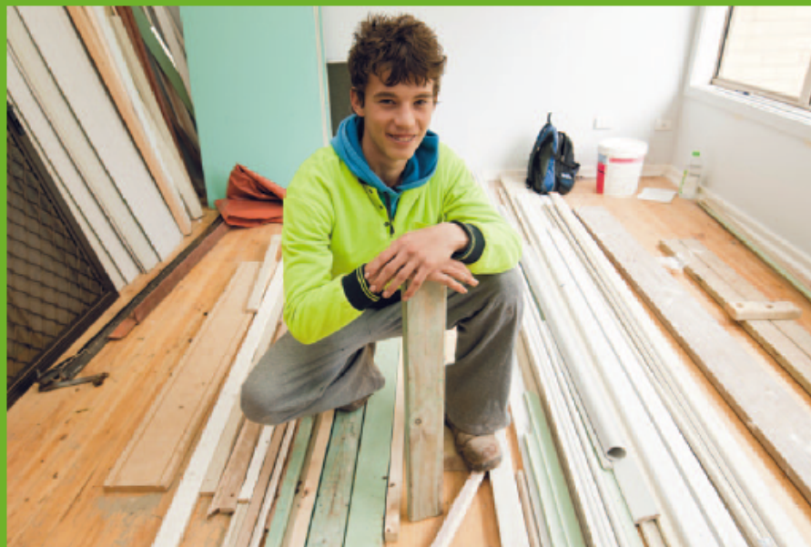
Brad Martin at work on a Zenith home renovation.
